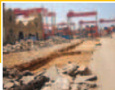
Construction of Container Stacks
