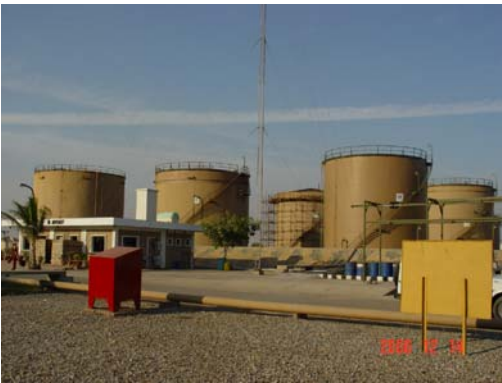
Tank Farm Area
