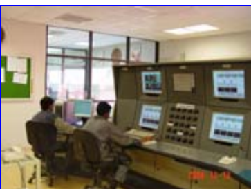
APC for Crude Unit
